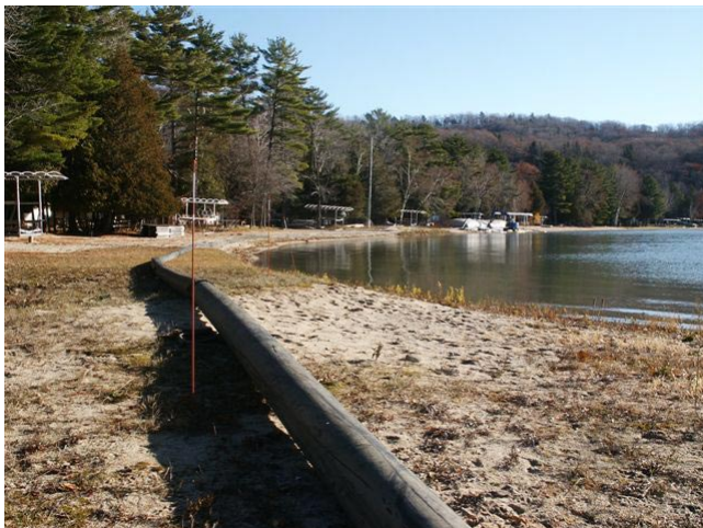
Pipe from dredger to sand drainage bag
