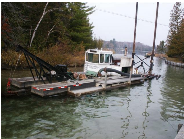
Hydraulic Dredge in the channel
